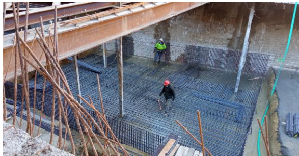
Figure 6 Preparation of the mat foundation solution.
