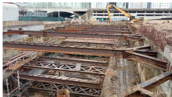
Figure 4 Metallic struts applied in site.
